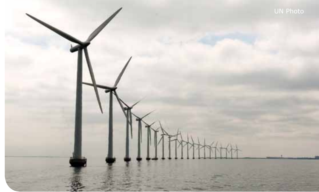
Middelgrunden offshore wind farm in Denmark
